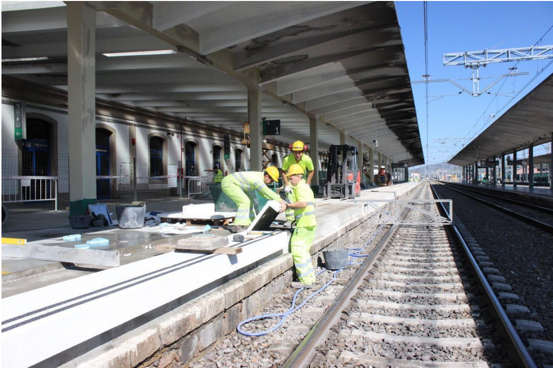
Figure 12. Modifications to platforms
