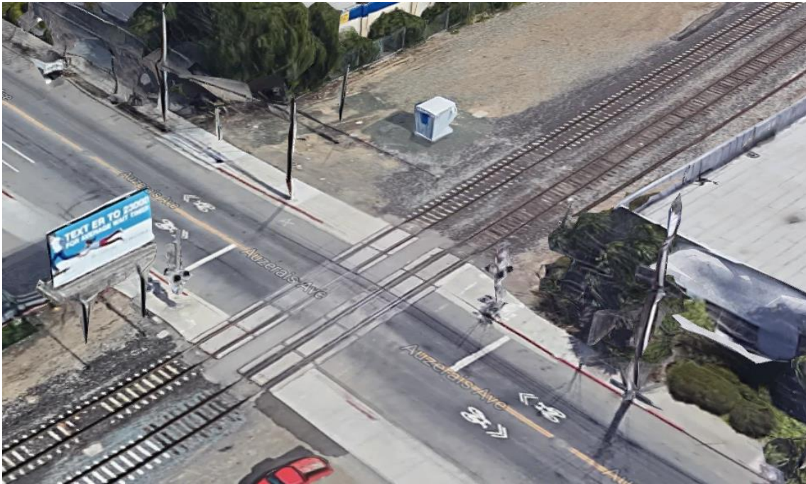
Figure 13. Typical at-grade crossing in railway line San Jose to Gilroy
