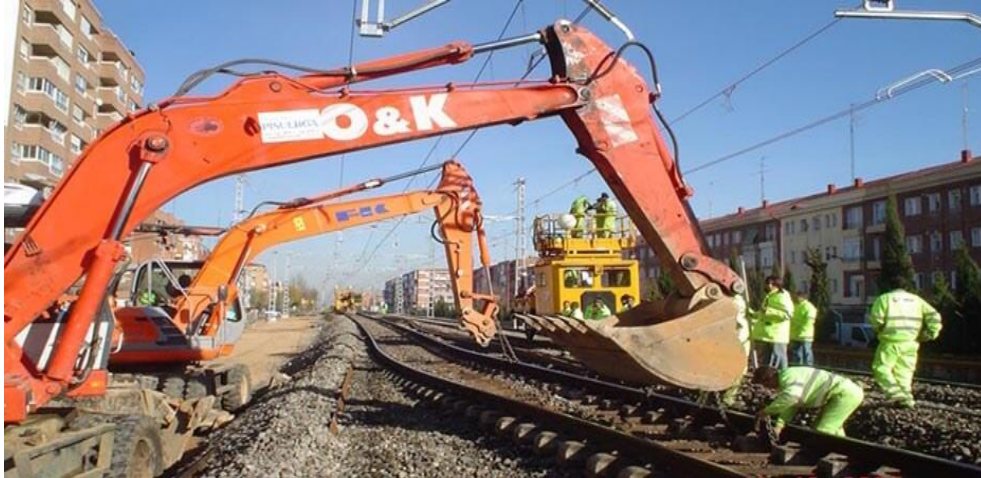
Figure 2. Lateral Displacements of the track between 1 and 10 ft
