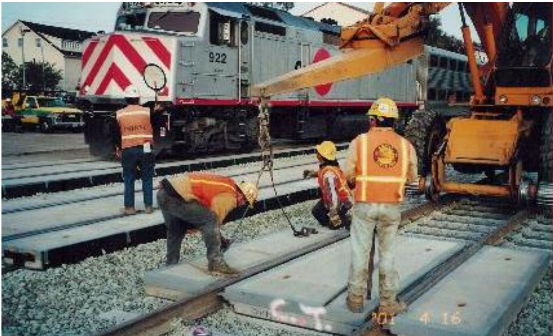
Figure 14. Construction of at-grade crossing
