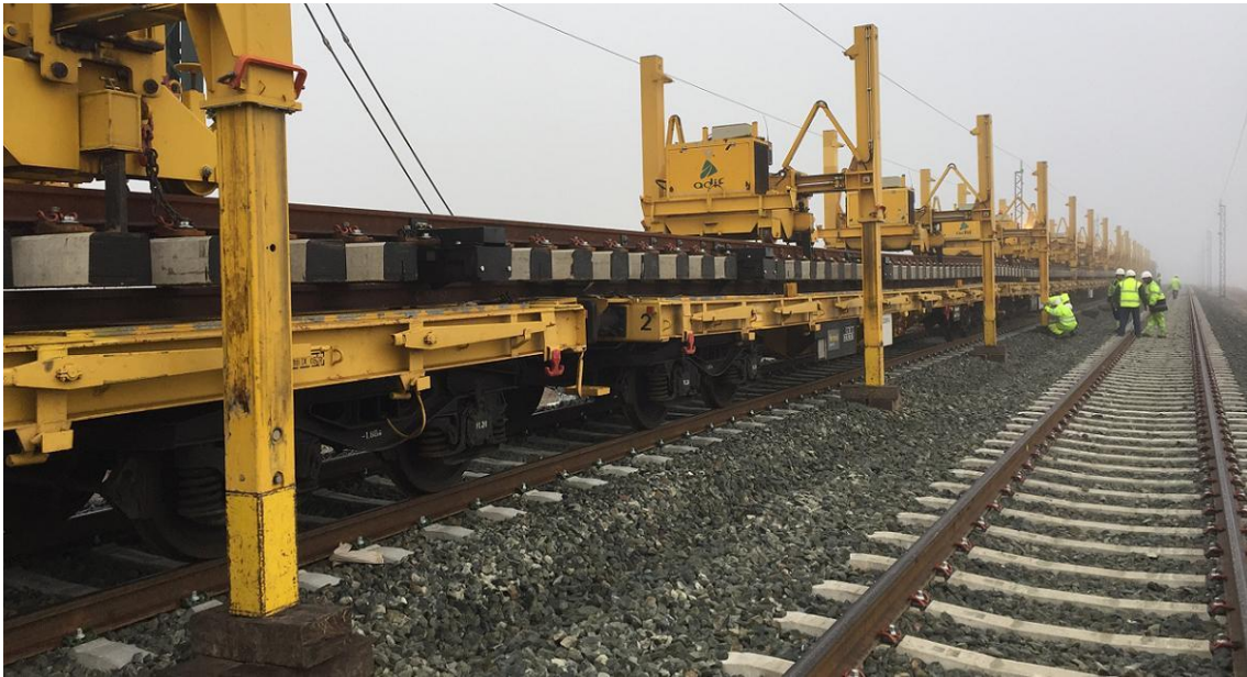
Figure 10. Transportation of a pre-assembled turnout
