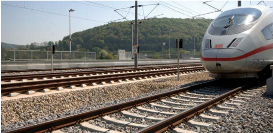
Figure 5-5 Ballast Track - Schotteroberbau
