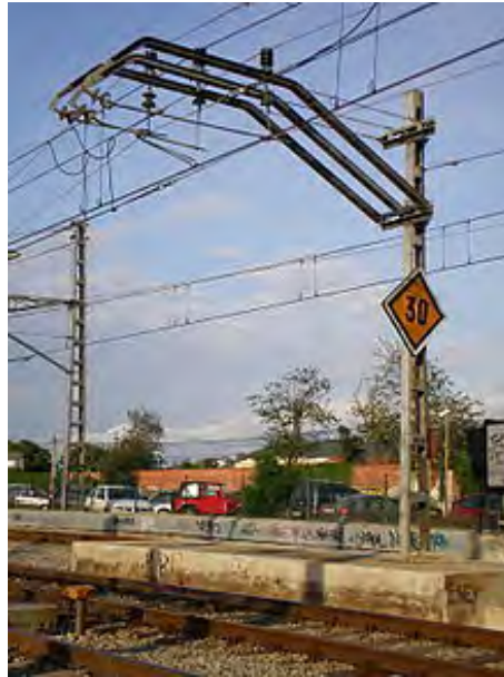
Figure A1-8. OCS temporary foundation
