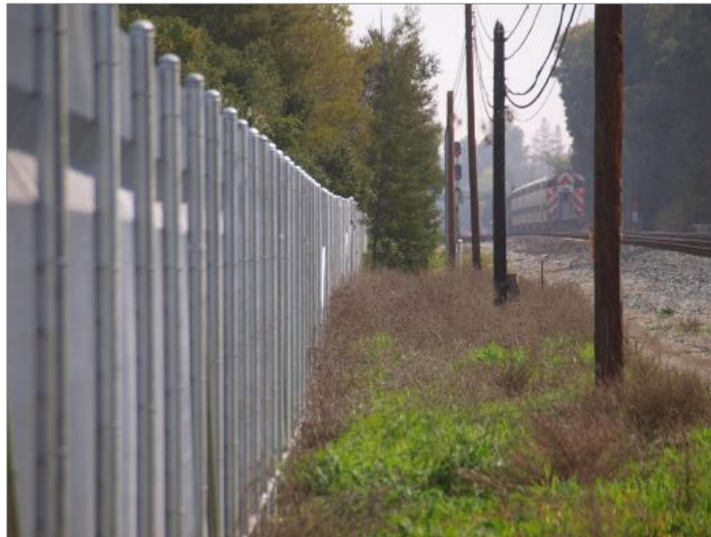
Figure 2-17 Photograph of Perimeter Fencing of Right-of-Way
