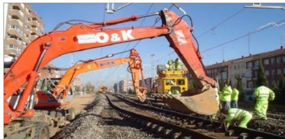
Figure 2-52 Construction of Lateral Track Shifts (<10 feet)
