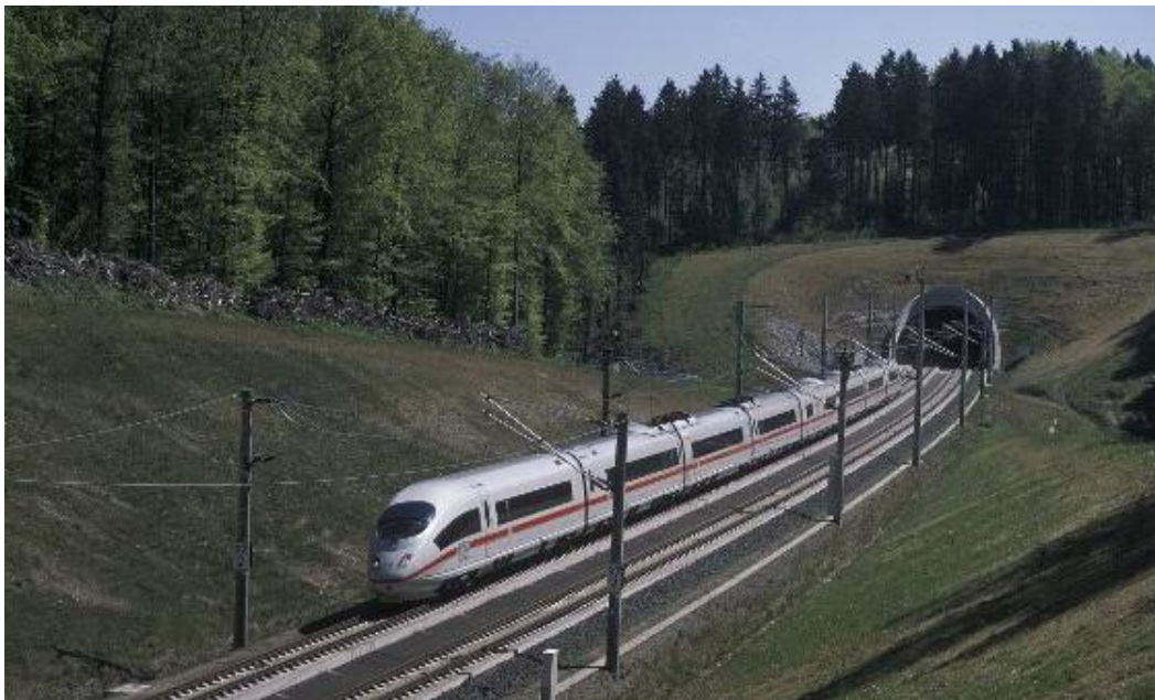
Figure 2-9 HST Emerging from Tunnel
