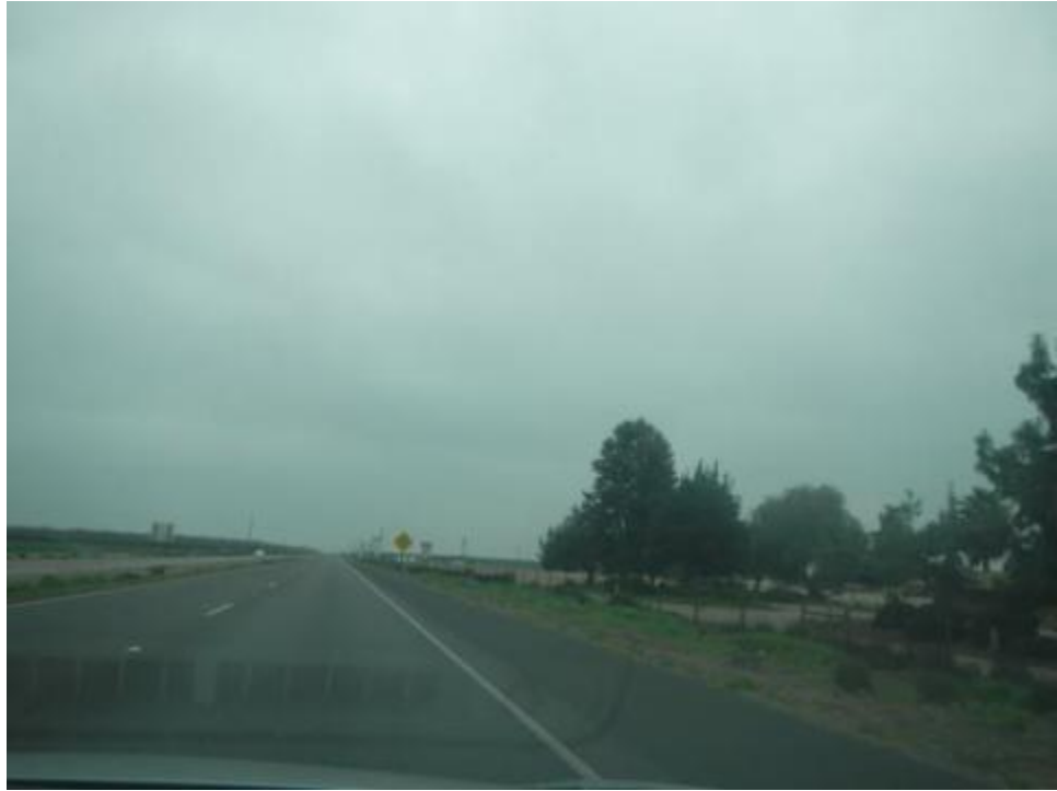
Photograph 9 View of SR 152 Looking East
