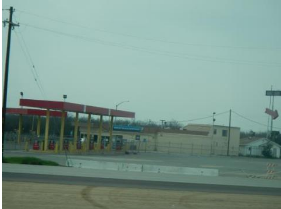
Photograph 17 View of Diesel County Truck Stop Facility along SR 99
