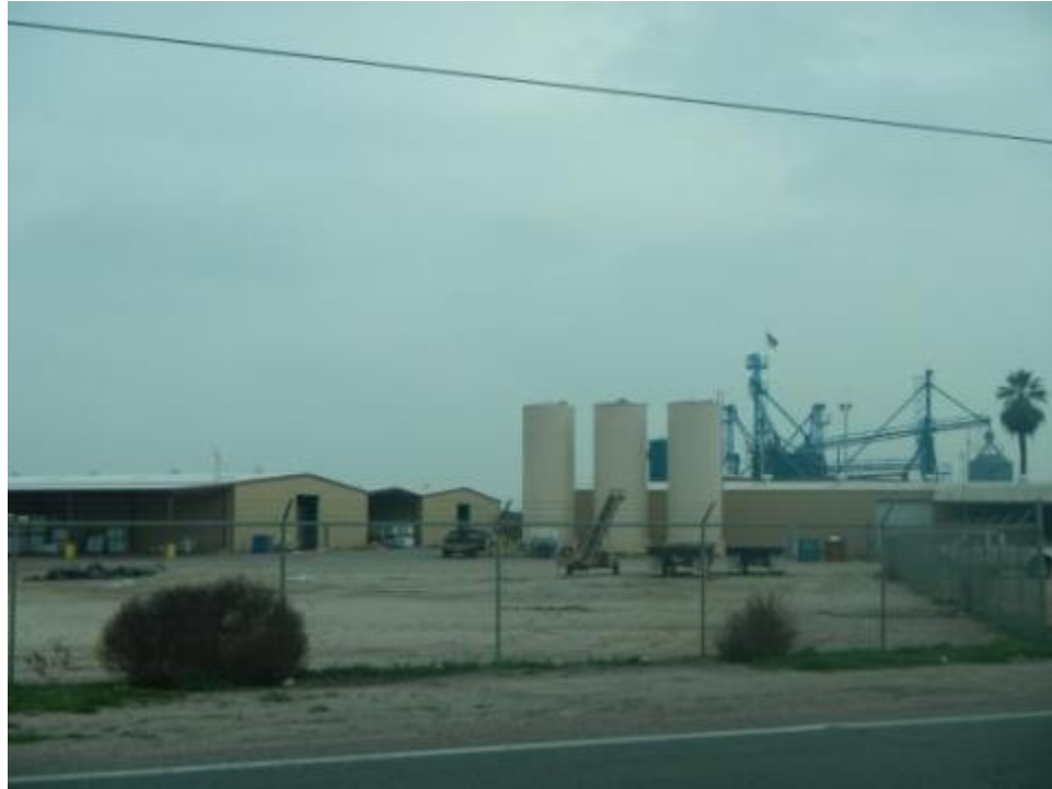
Photograph 15 View of the Lockwood Seed Company Facility
