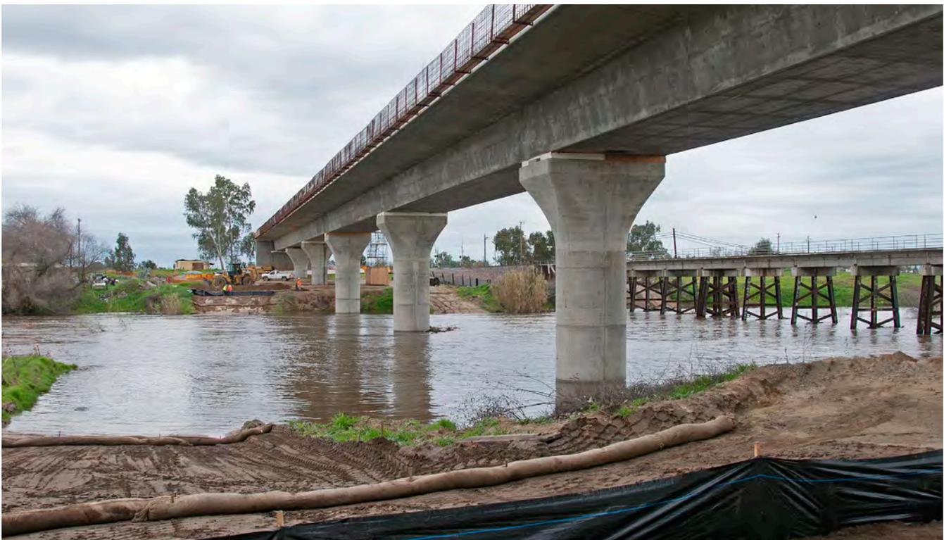
**PHOTO:** The Fresno River Viaduct maintains clearance beyond the main river channel to maximize movement along this important wildlife corridor.
