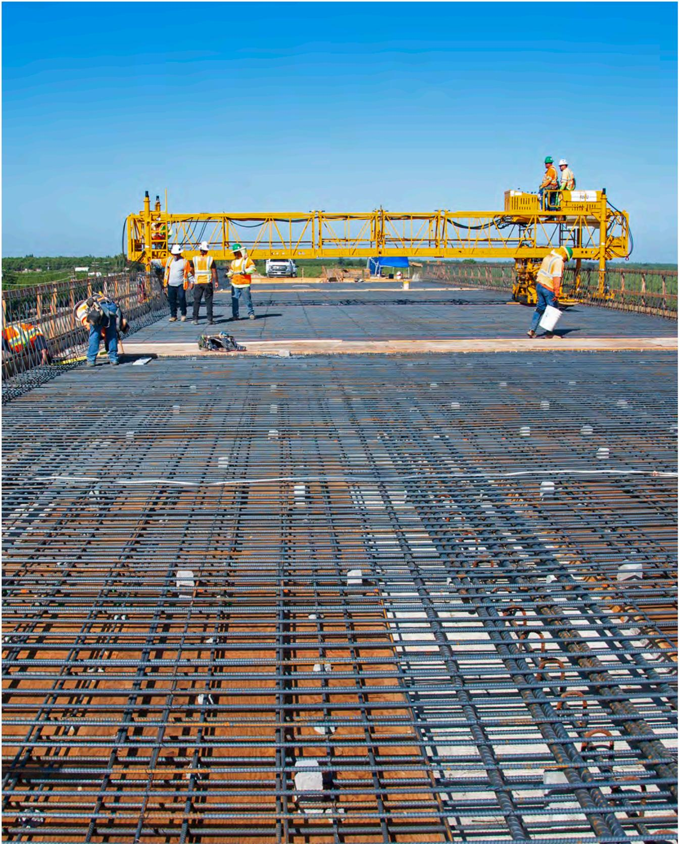
**PHOTO:** This Tier 4 gantry is being used at the Excelsior Avenue grade separation.
