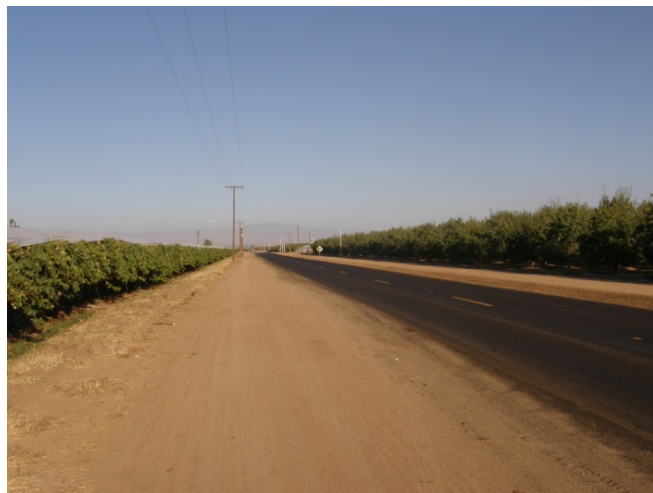
V-c. F-B LGA at vineyard and orchard on Burbank Street, looking east
