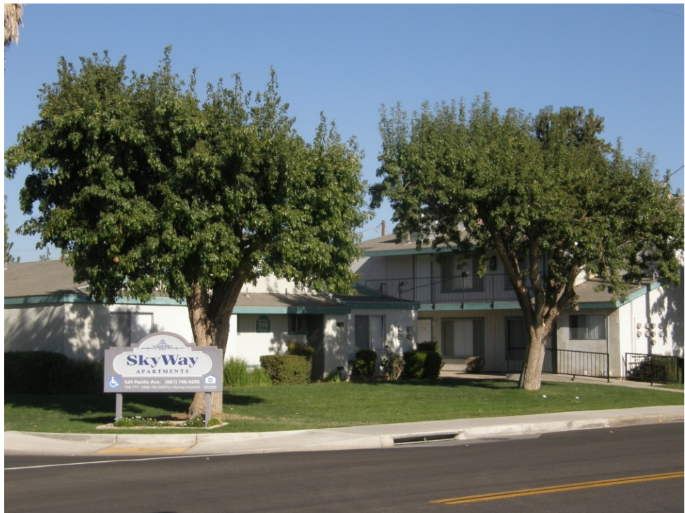
SR-b. Multifamily apartments southeast of Walker and State Streets
