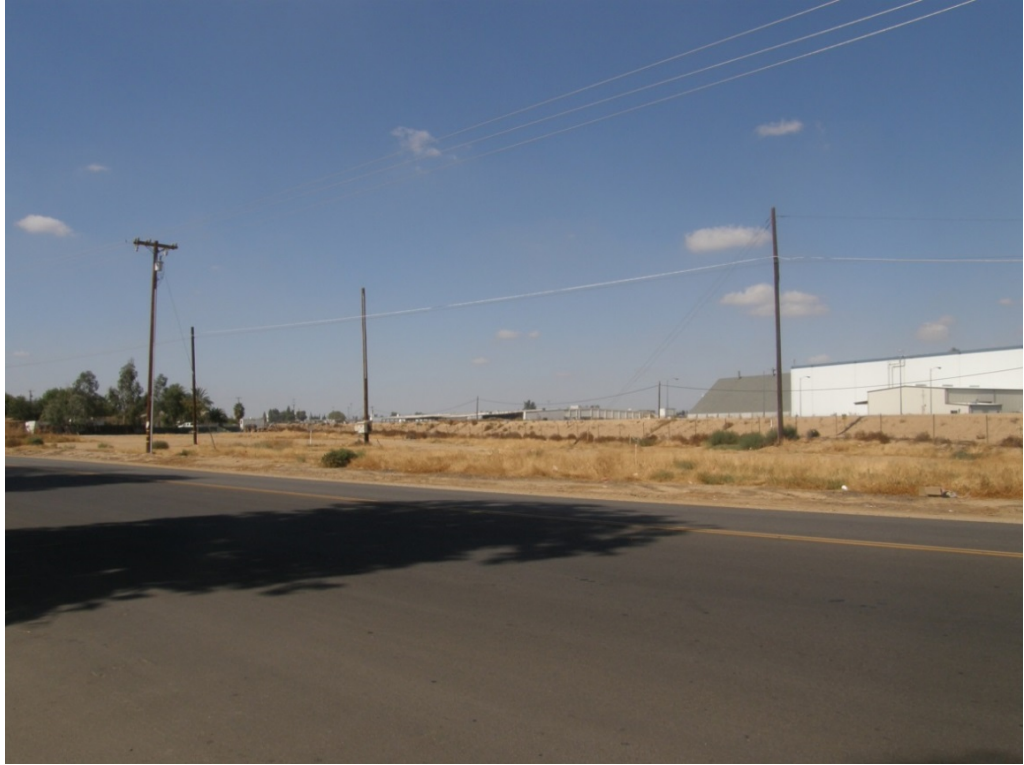
NBR-a. View of F-B LGA north of multifamily residences on Norris Road
