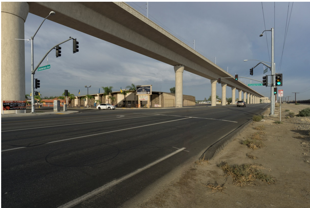
KVP 12. Simulated view of Mercado Latino Tianguis in east Bakersfield looking west from Edison Highway
