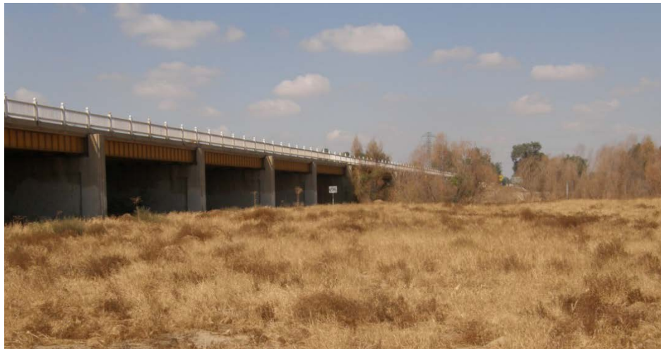
KR-b. F-B LGA at Kern River, looking west from Kern River Parkway Bike Trail
