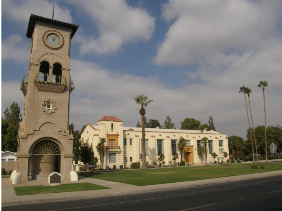
CBI-a. Kern County Museum on Chester Avenue to north of proposed 34th Street entrance to Bakersfield F Street Station, looking west
