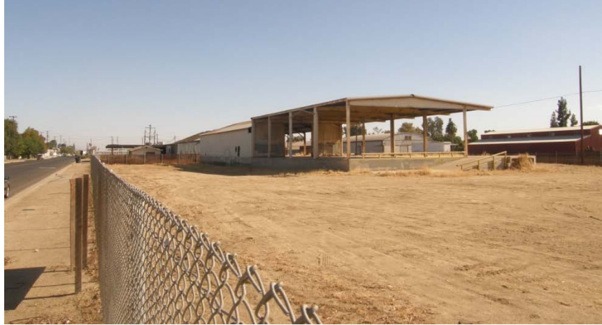
SC-a. Alignment at vacant business park along BNSF Railway, looking south
