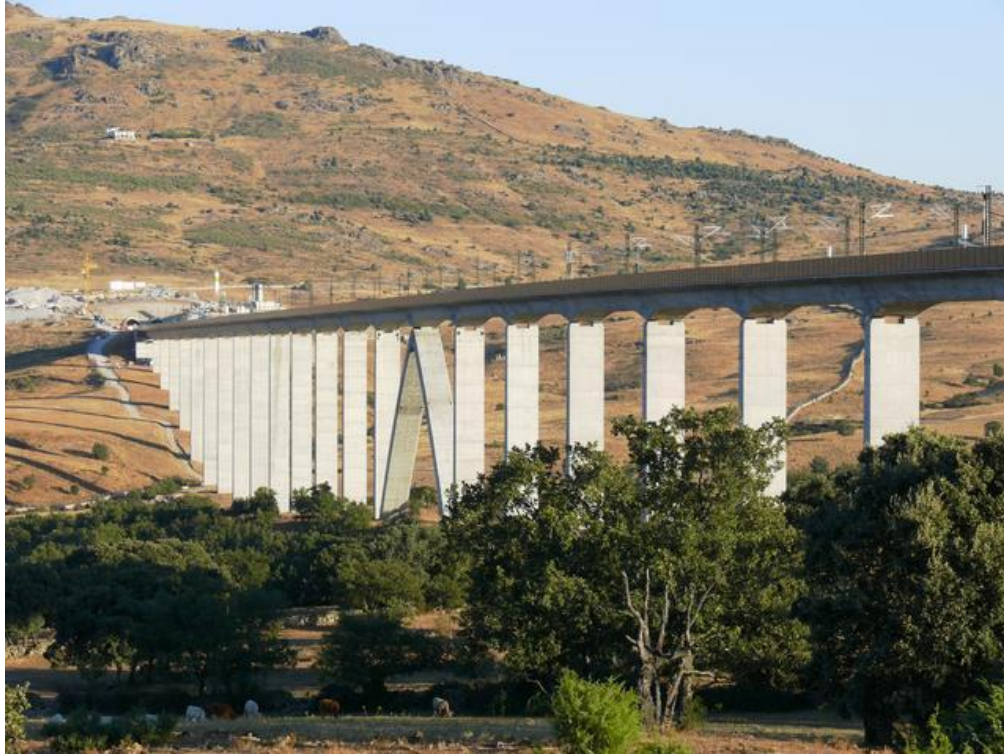
Figure 3-6: AVE High Speed Rail Viaduct
