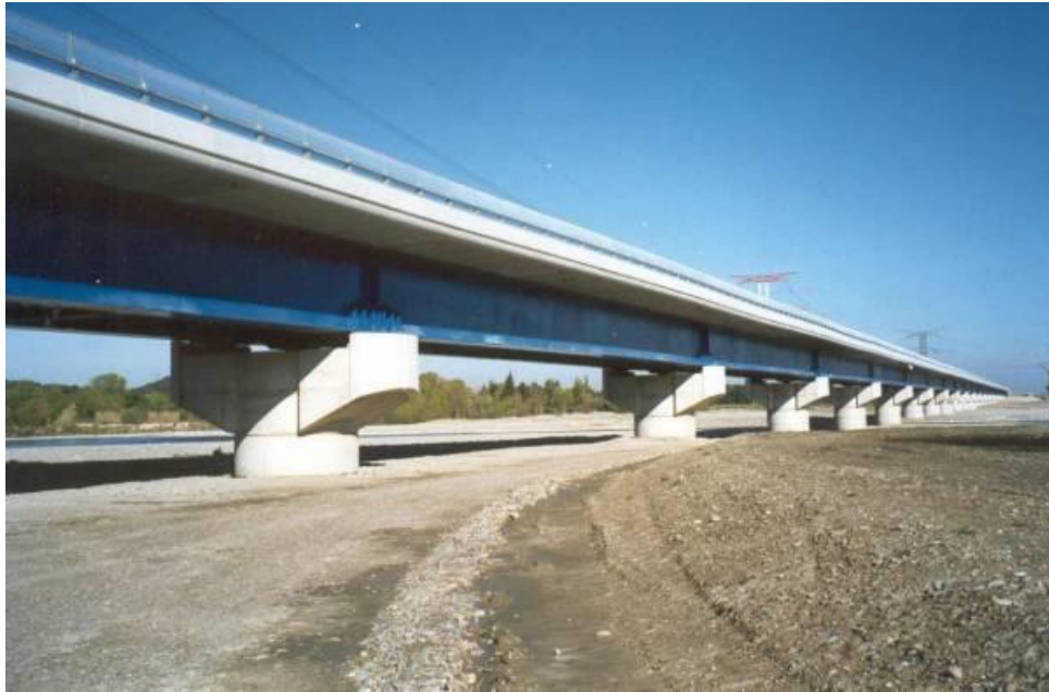
Figure 3-3: Cheval Blanc Viaduct, France
