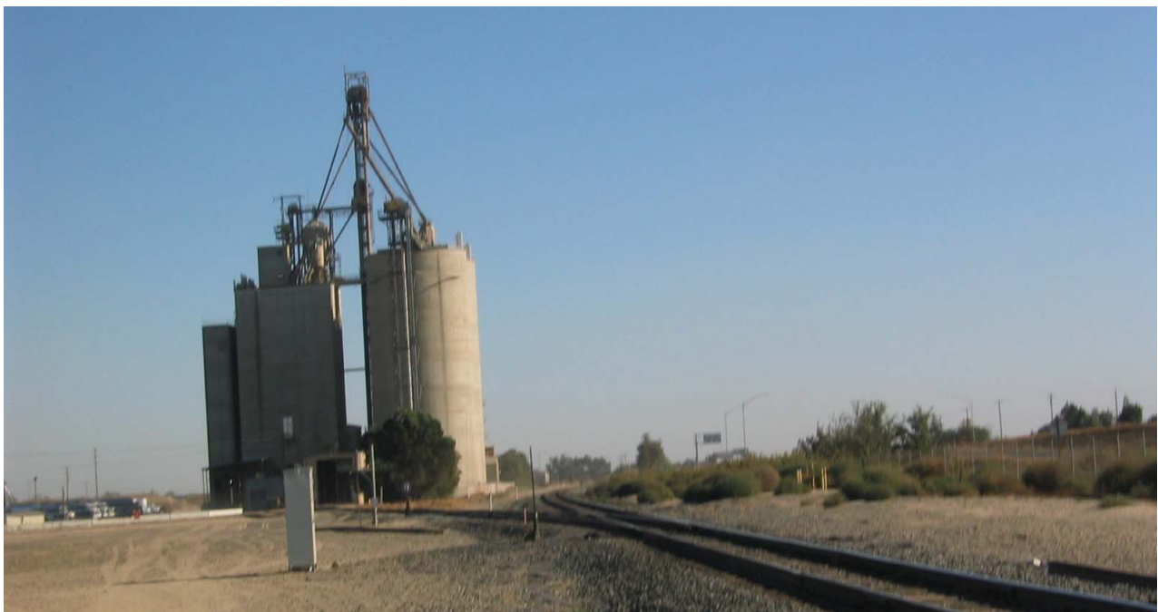
Figure 4-6 Spur Serving Large Silo along UPRR
