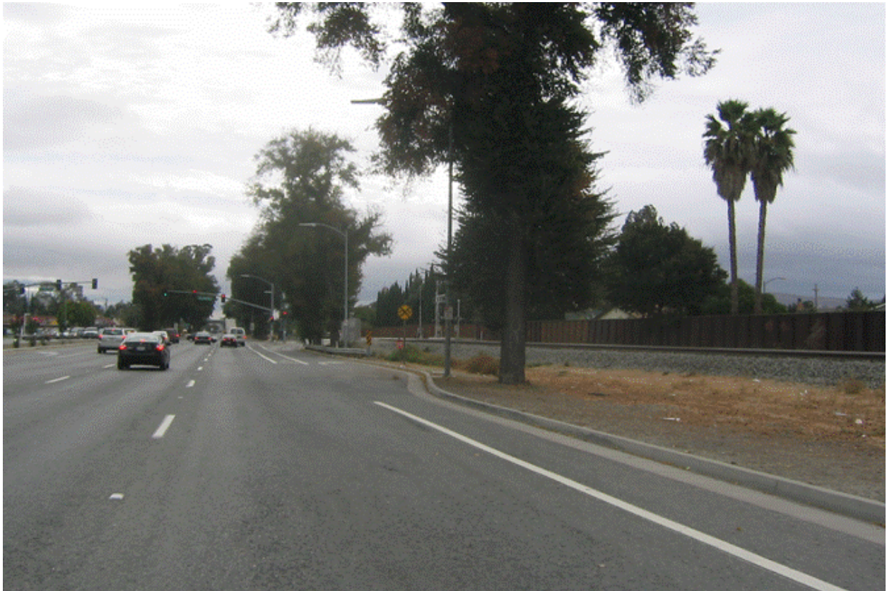
Figure 2-1 Revised Figure 3.9-11—Caltrain/UPRR along Monterey Highway (May 2008)
