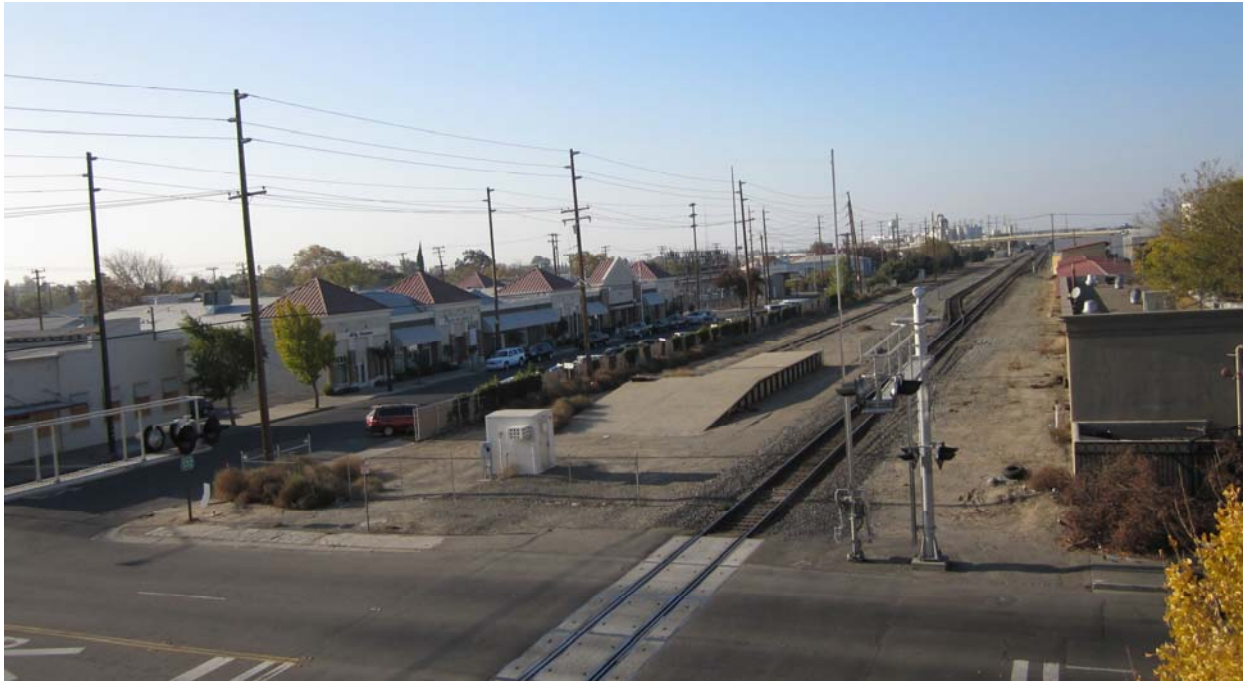
Figure 4-7 Typical Team Track Facility
