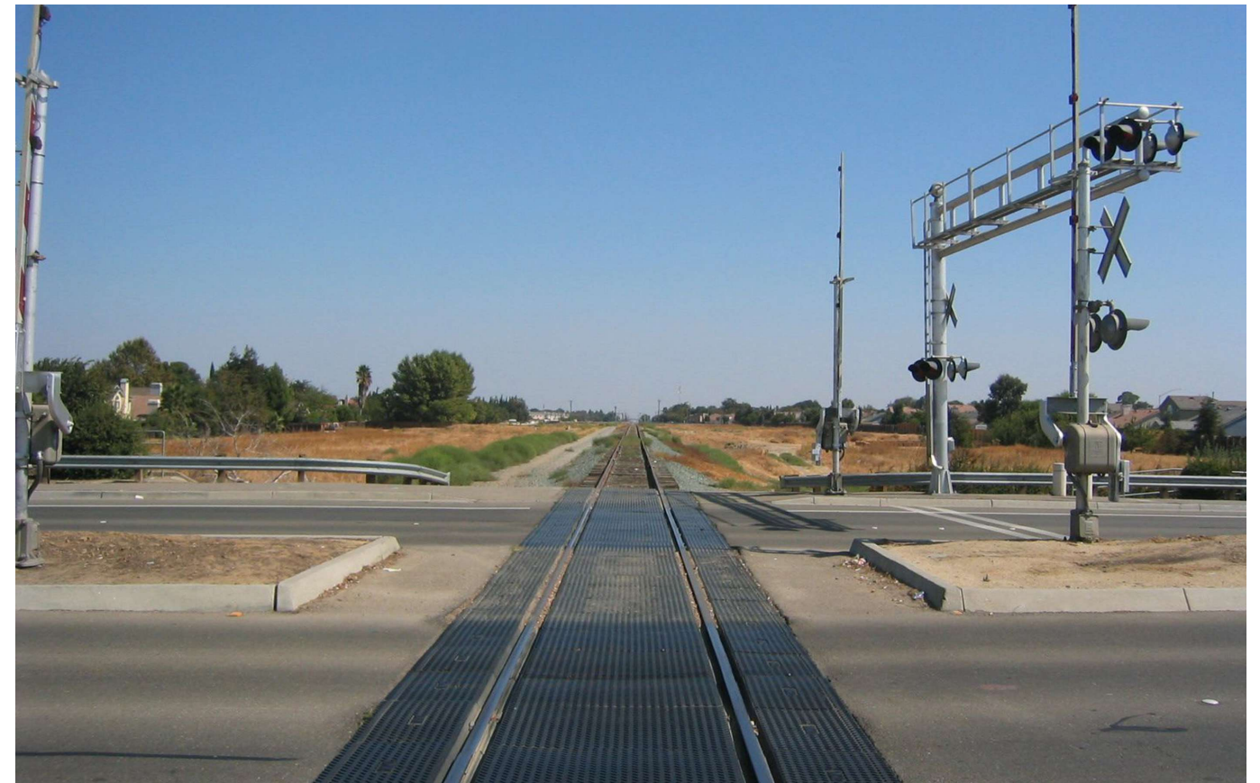
The cross section shown below shows that the HST would be elevated over the roadway pictured above.
