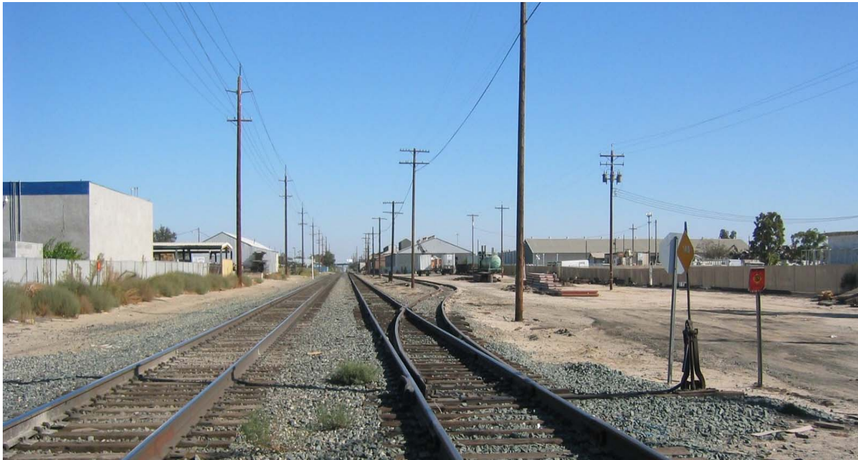
Figure 4-1 Typical Spur Track or Siding
