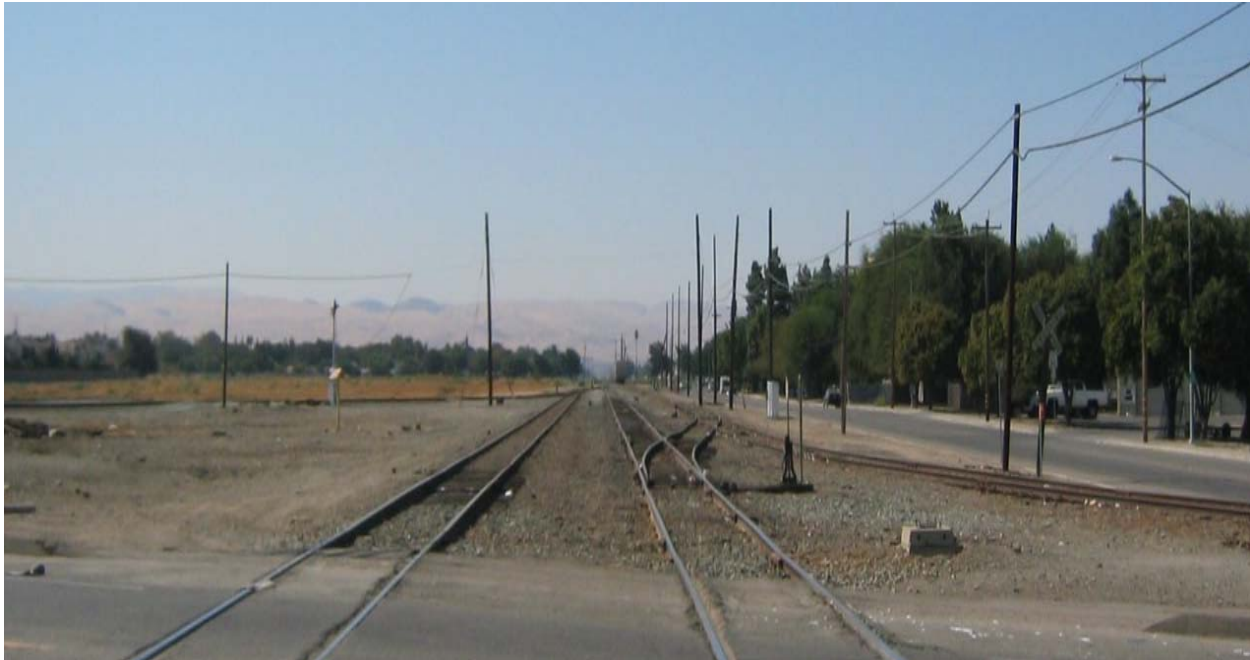
Figure 4-4 Westside Branch Junction in Tracy
