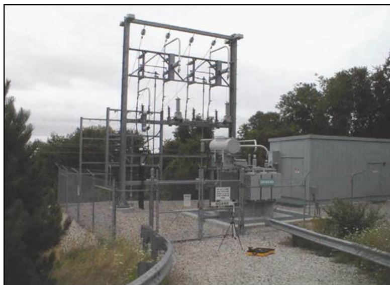
Figure 2-27 Paralleling Station
