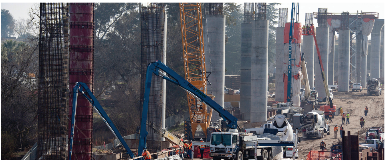
San Joaquin River Viaduct Construction in Fresno
