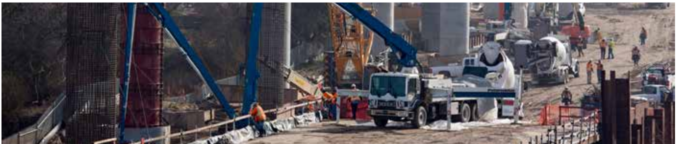
San Joaquin River Viaduct Construction in Fresno
