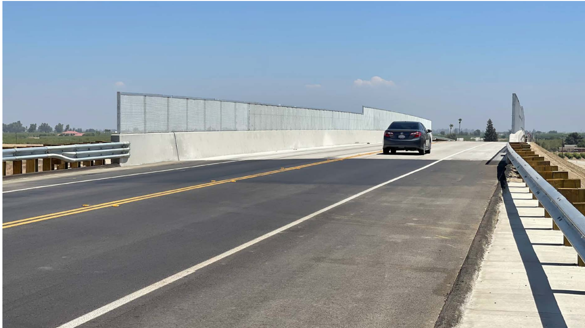
The Mountain View Avenue Grade Separation is now open and takes traffic safely over the existing railroad and future high-speed rail tracks.
