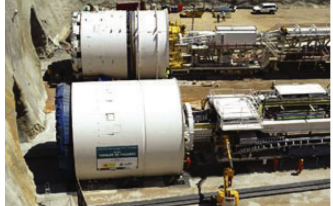
Tunnel boring machines constructing a dual-bore tunnel.
