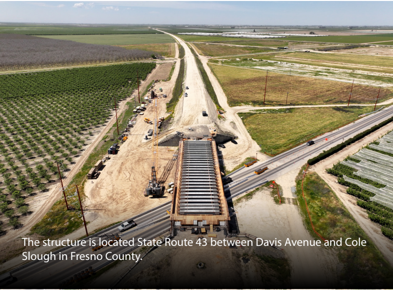
The State Route 43 Tied Arch Bridge will take high-speed trains over State Route 43.
