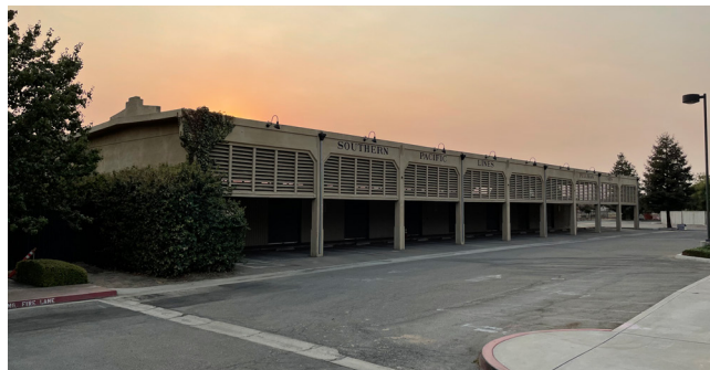
Historic Fresno Train Depot Pullman Shed.
