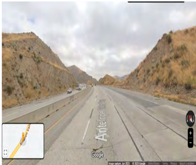
Figure 2. Looking north at the steep cut slopes along the SR 14 freeway adjacent to Bee Canyon.
