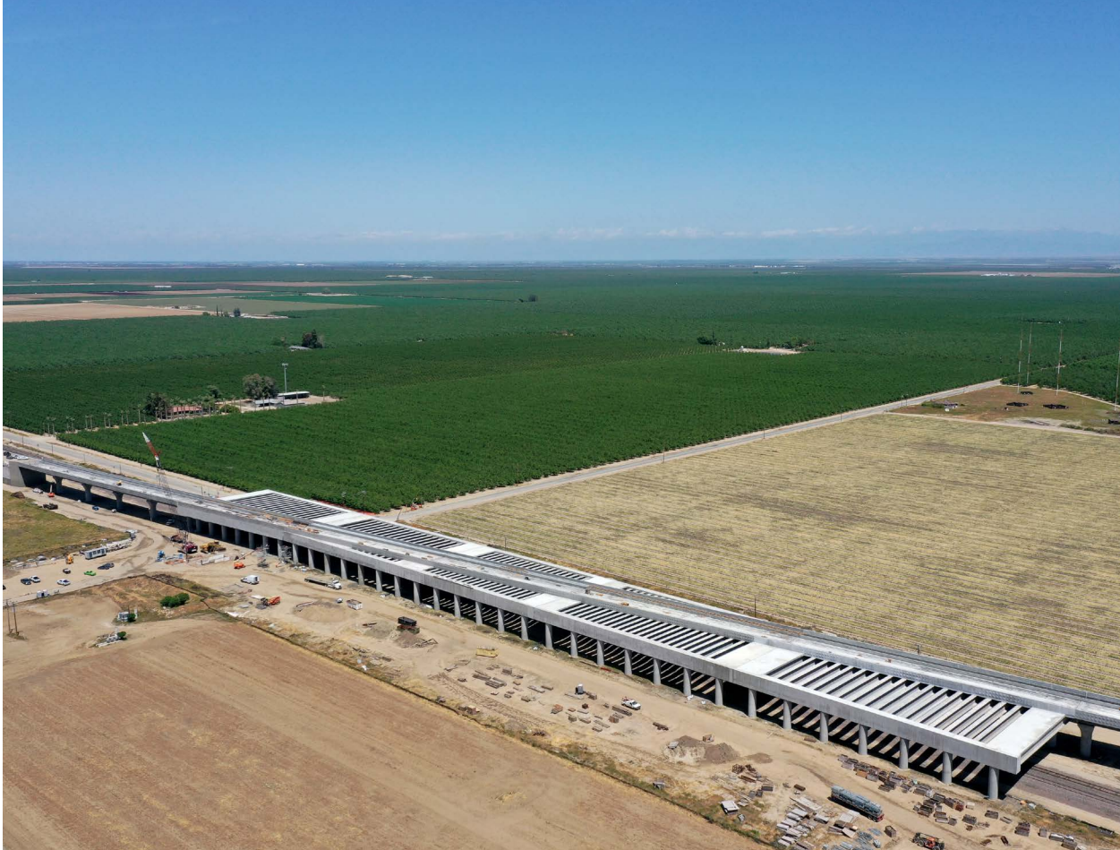
Photo: Wasco Viaduct in Kern County
