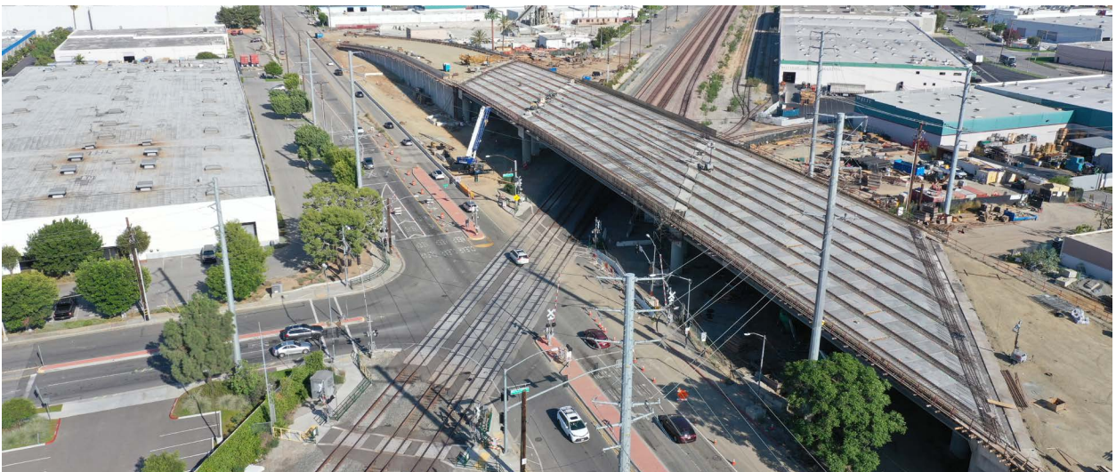
Photo: Rosecrans Avenue and Marquardt Avenue grade separation (under construction)
