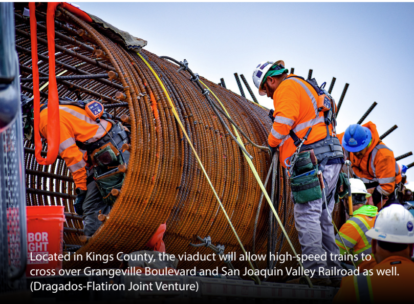
Workers unloading a rebar cage at the Hanford Viaduct. (Dragados-Flatiron Joint Venture)
