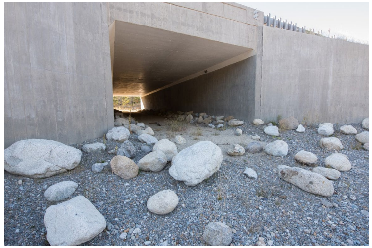
Figure 3. Typical Wildlife Undercrossing
