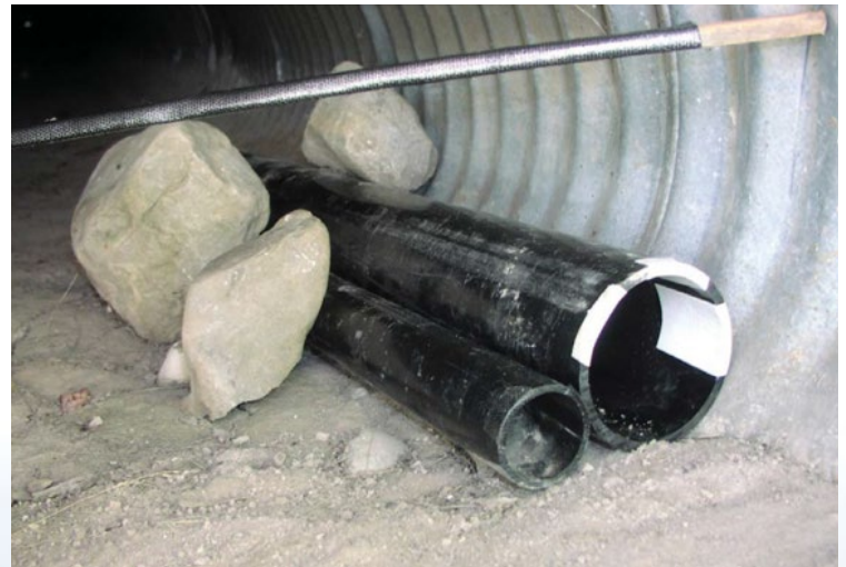
Figure 4. Dual Purpose Culvert/Wildlife Undercrossing
