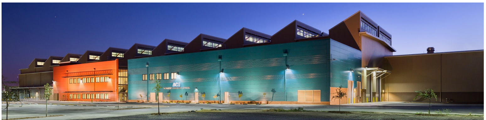
Example of a modern rail maintenance facility: Stockton's LEED® Silver ACE train maintenance facility opened in 2015. (Photos: San Joaquin Regional Rail Commission)
