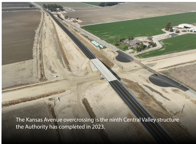
The structure required 1,300 cubic yards of concrete and 334,000 pounds of rebar to complete.
