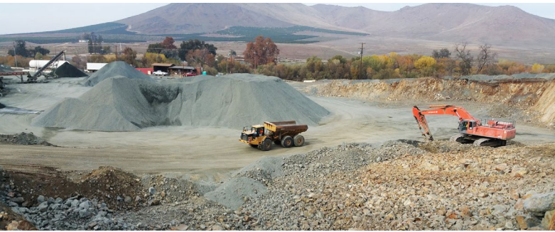
Deer Creek Rock and Asphalt Facility in Porterville, CA (Jaxon Enterprises)
