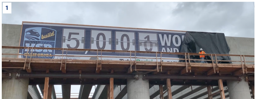
1. It's hard to miss the huge banners that recently went up on high-speed rail structures in the Central Valley touting more than 5,000 jobs created since construction began on the high-speed rail project. Dumont Printing of Fresno manufactured the signs celebrating that milestone.
