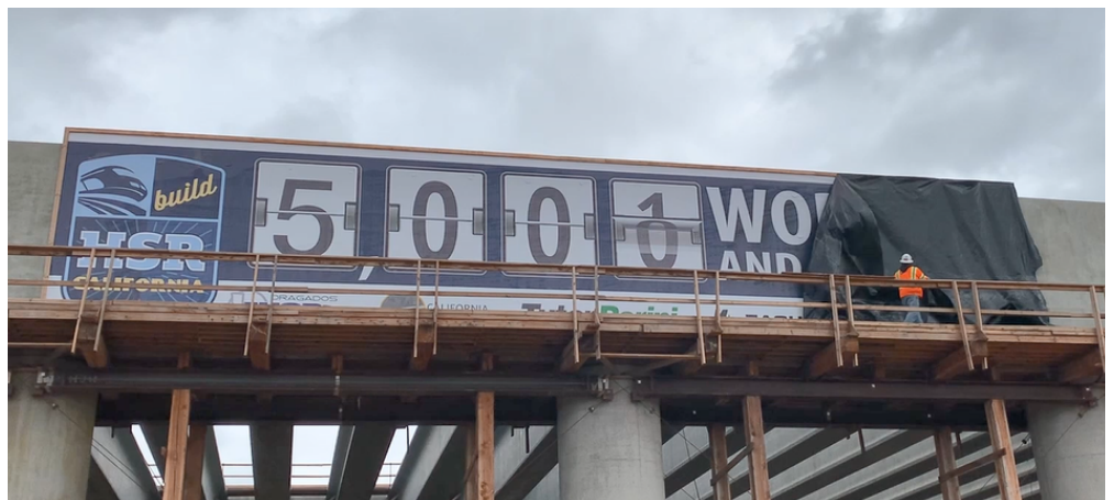
In February, crews unveiled new banners on the Cedar and Wasco Viaducts. They are part of the Authority's celebration of 5,500 jobs created since high-speed rail construction began in the Central Valley. More jobs are being added every day. Most of the construction workers on those jobs hail from the Central Valley.
