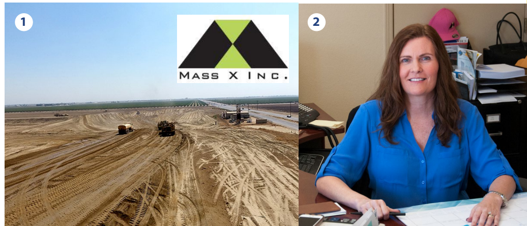
1. Mass X Inc. crews move a massive amount of dirt and make sure it will support a two-and-a-half-mile-long embankment that will carry high-speed rail trains just south of Fresno near American and Cedar Avenues. 2. Mass X owner Jennifer Foster said, "High-speed rail has been a good opportunity for our small business. It's keeping our employees working on a ground-breaking project that is local, and this may open the door for future work on the project."
