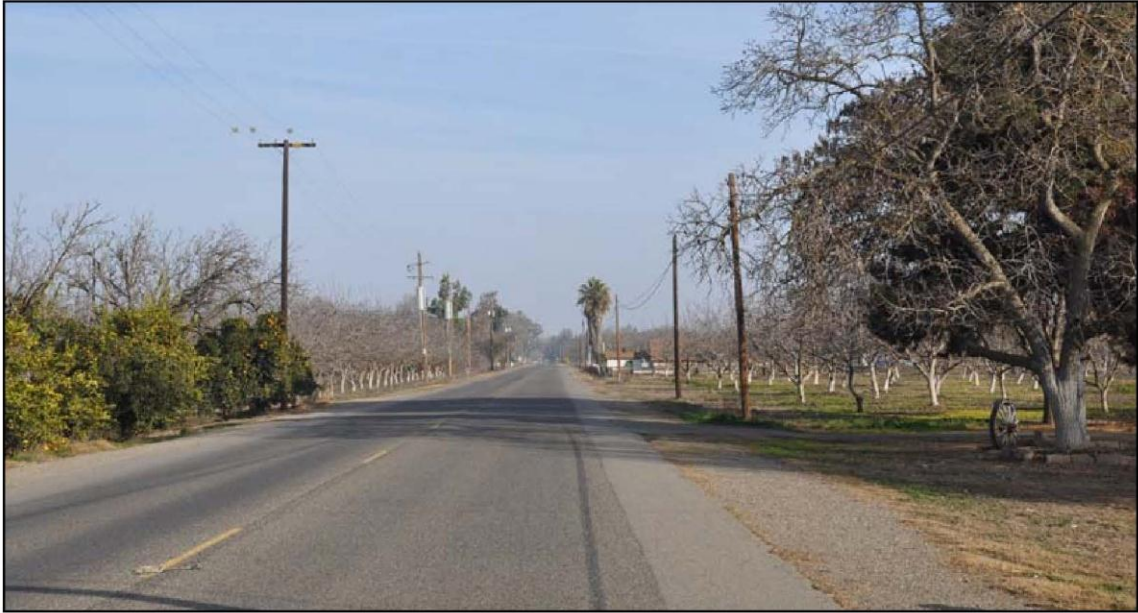
a. Existing View
