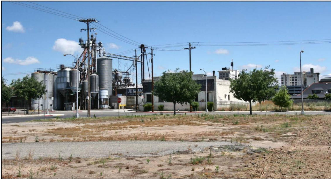
RI-b. View from China Alley near Mariposa Street, looking north toward alignments.
