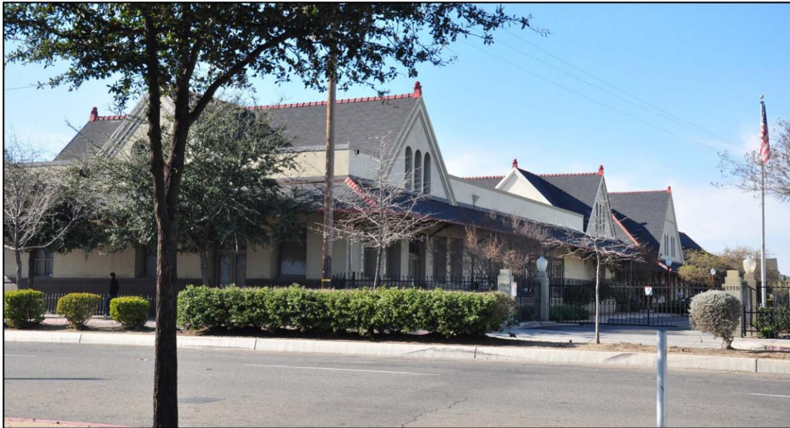
CBD-d. Southern Pacific train station, looking west from Tulare and H Streets
