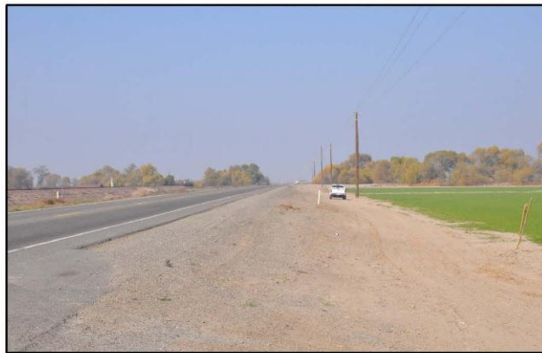
VR-b. Alignment crossing at Tule River from Highway 43.
