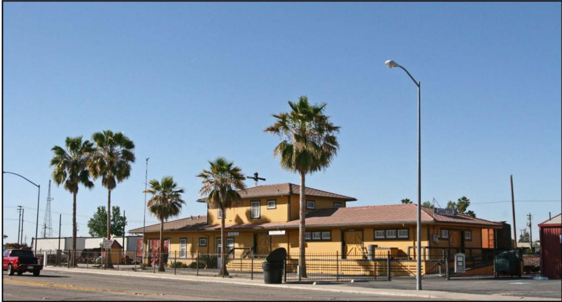
a. Existing View
