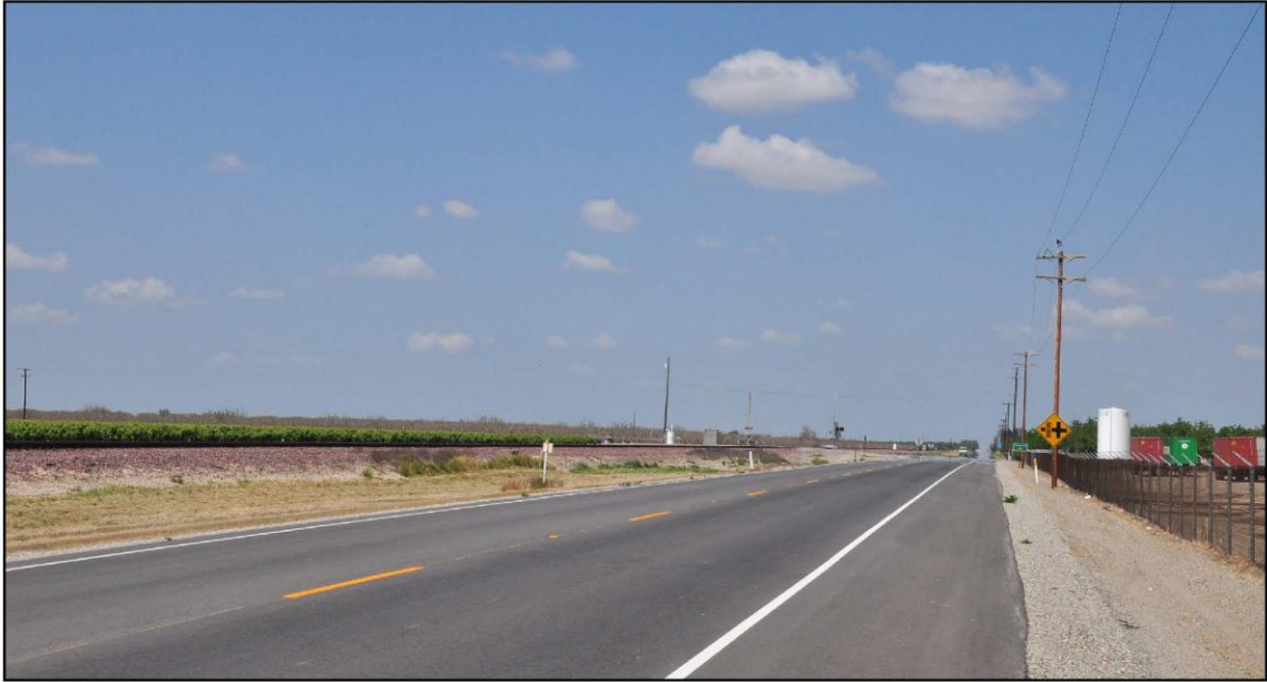
a. Existing View
