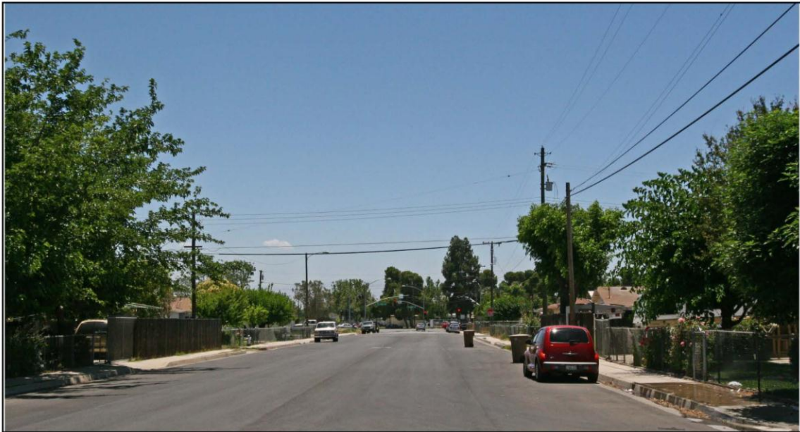
EBR-b. Bakersfield South alignment from Owens St., looking south.
