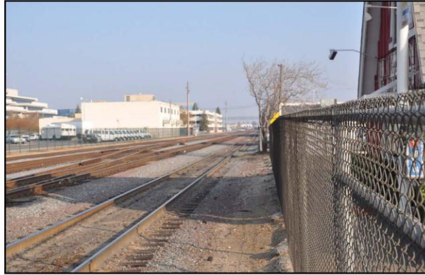
CBI-a. Project alignments looking east near Chester Avenue, downtown Bakersfield.
