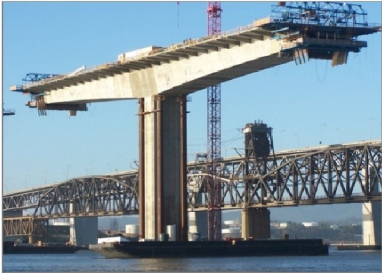
Figure 2-100 Balanced Cantilever Segmental Construction
