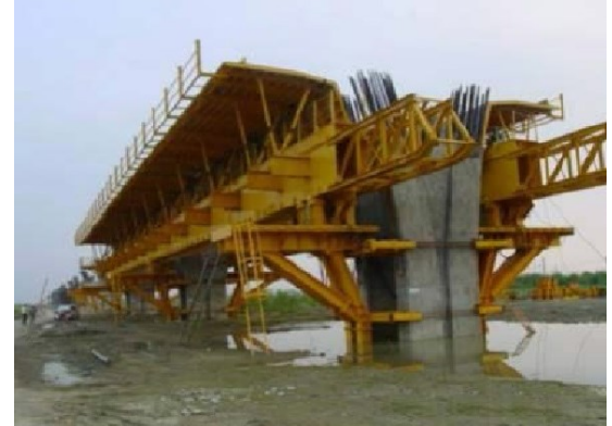
Figure 2-101 Cast-in-Place Construction on Falsework
