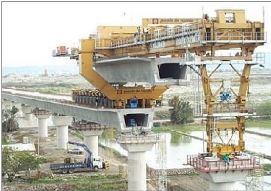
Figure 2-98 Full Span Precast Construction
