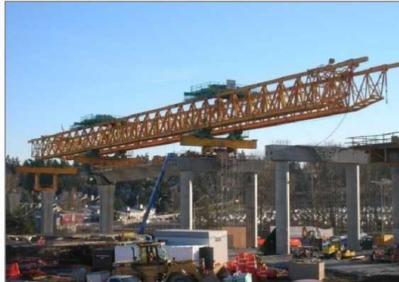
Figure 2-99 Span-by-Span Precast Segmental Construction
