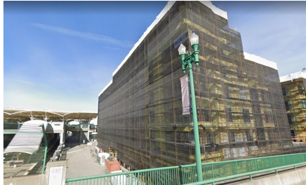
Gateway at Millbrae Station under construction
