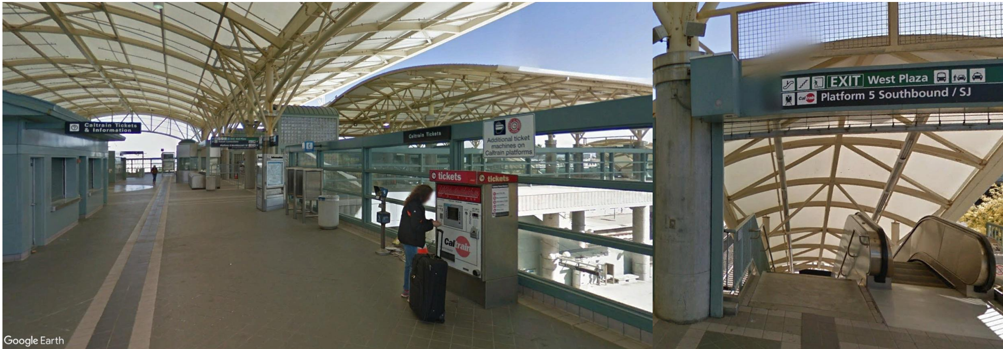
View of Concourse Level
