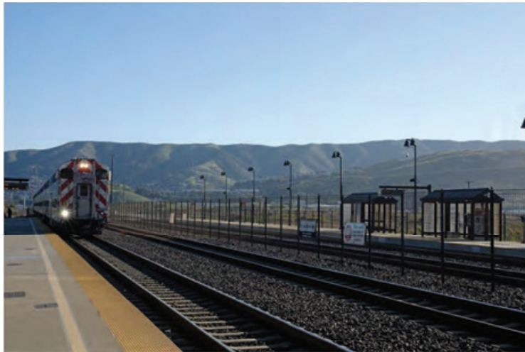
Figure Metis-16: Bayshore Caltrain station, March 2020.
