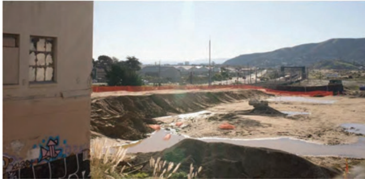
Draft EIR/EIS Figure 3.15-22: View of Bayshore Caltrain station from the Schlage Lock construction site.
