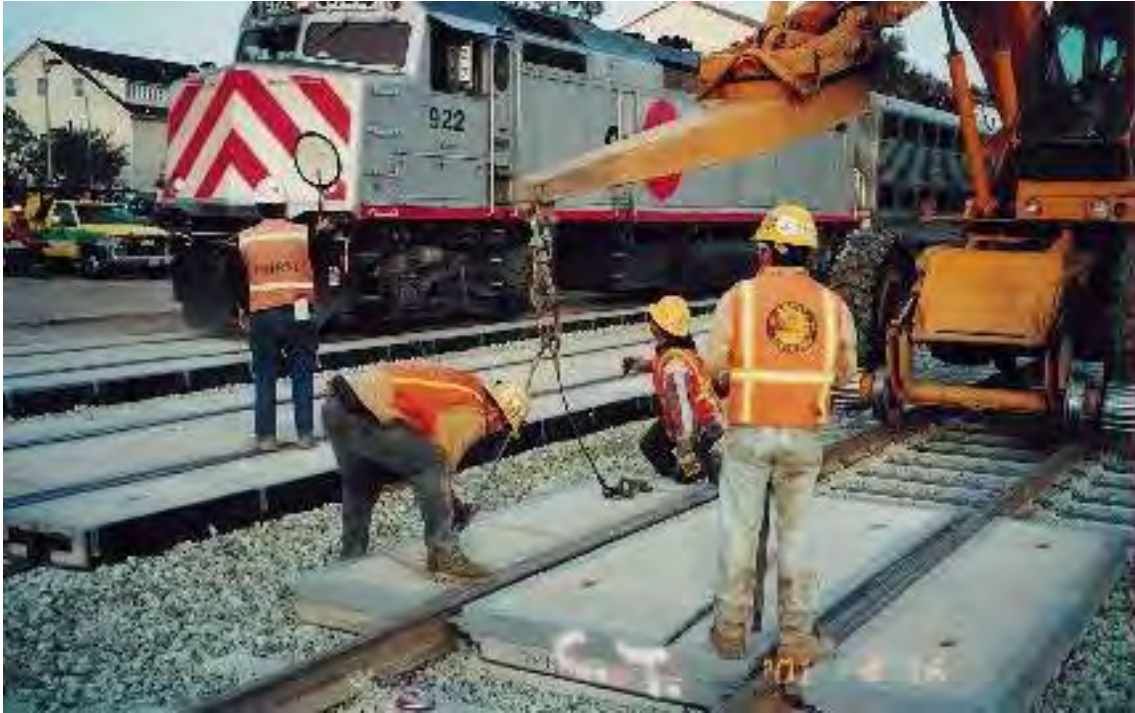
Figure 18. Construction of at-grade crossing
