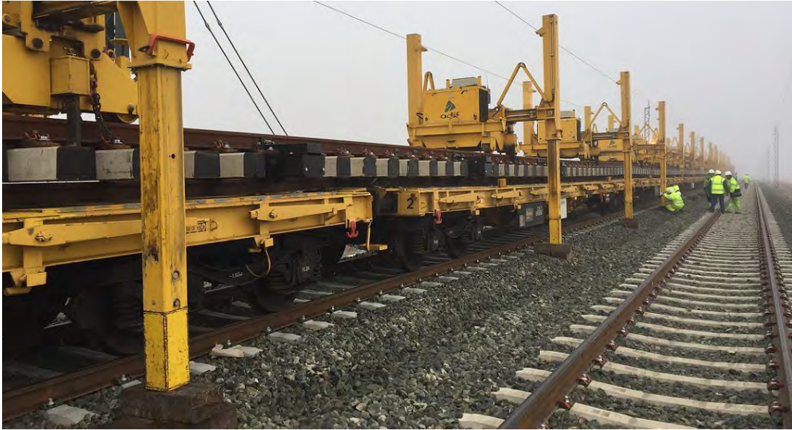
Figure 14. Transportation of a pre-assembled turnout
