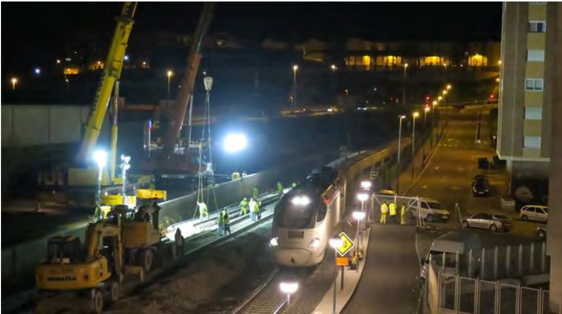
Figure 15. Assemble of a pre-assembled turnout with cranes
