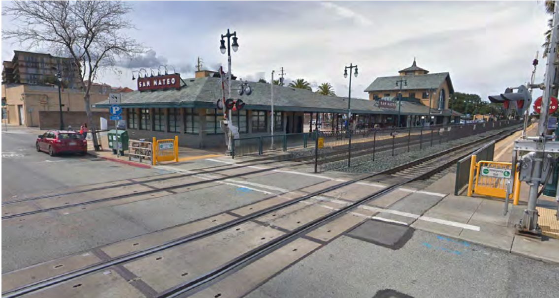
Figure 17. Typical at-grade crossing in railway line San Francisco to San Jose
