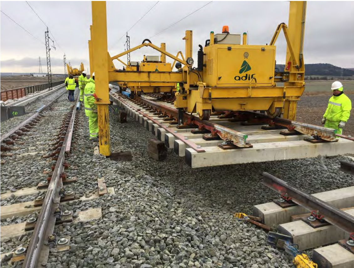
Figure 13. Assembly on the track of a pre-assembled turnout
