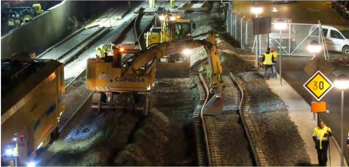
Figure 5. Lateral Displacements of the track greater than 21.34 ft
