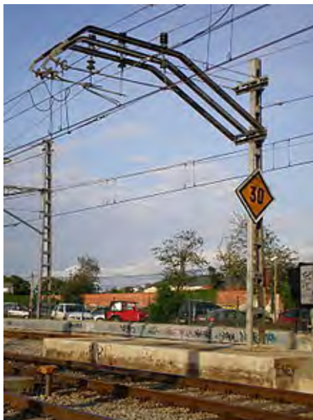
Figure A1-8. OCS temporary foundation
