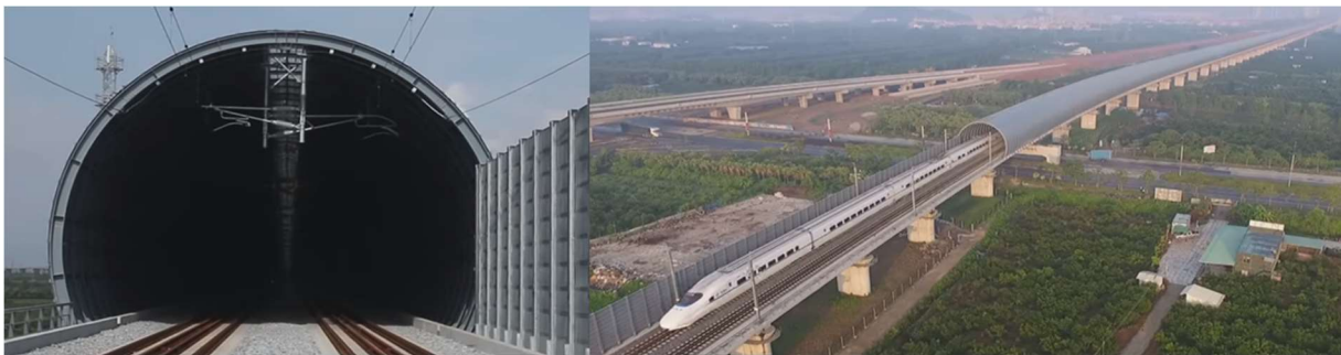
Figure 2: Shenzhen-Maoming Guideway Enclosure
