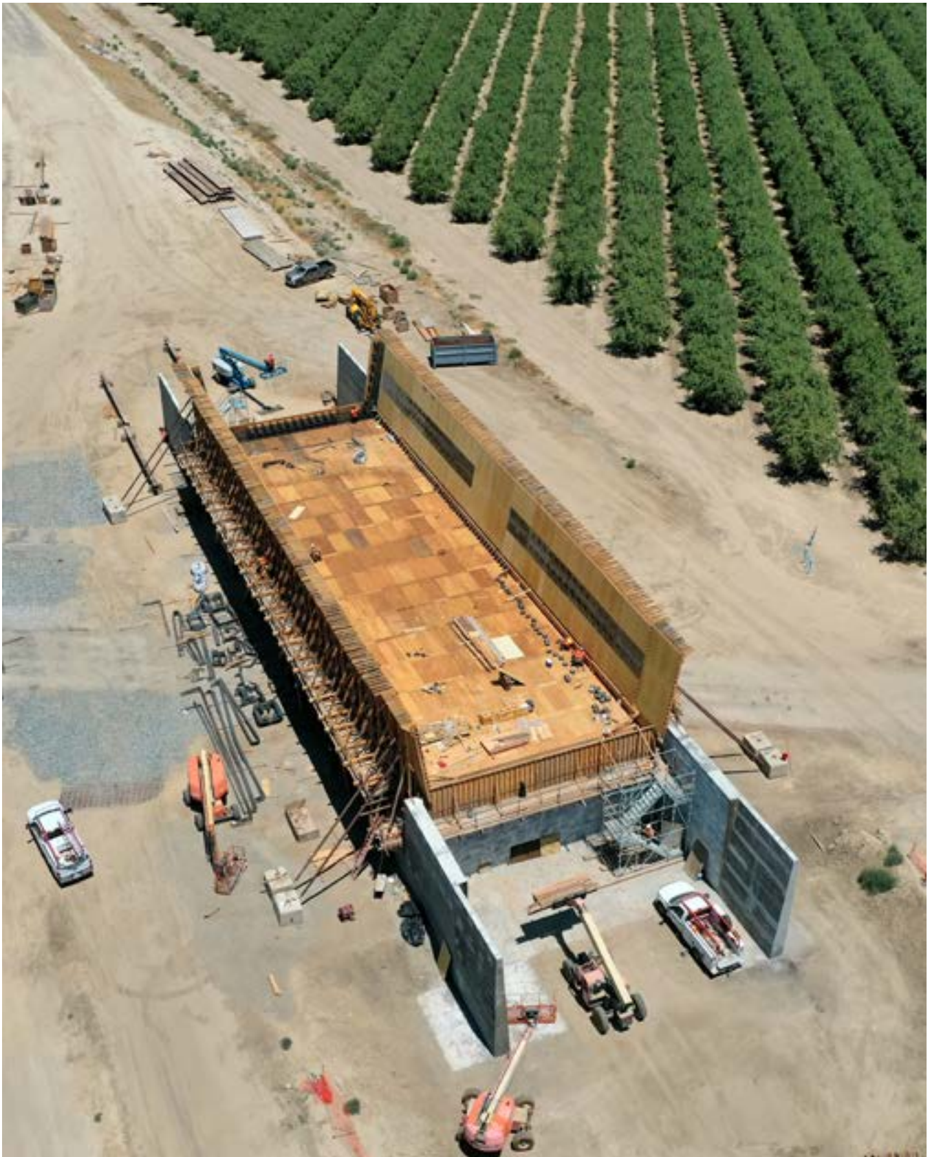
PHOTO: Work continues on Peterson Avenue viaduct construction in Kern County.
