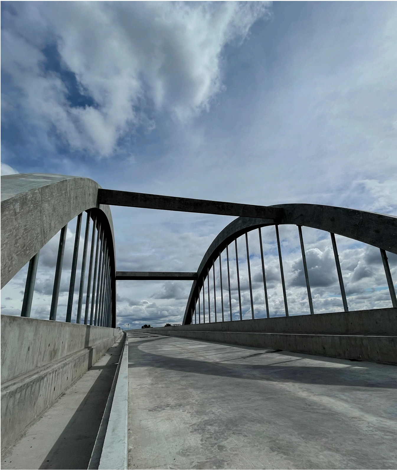
PHOTO: The San Joaquin River Viaduct’s highly visible arches represent the northern gateway into the city of Fresno.
