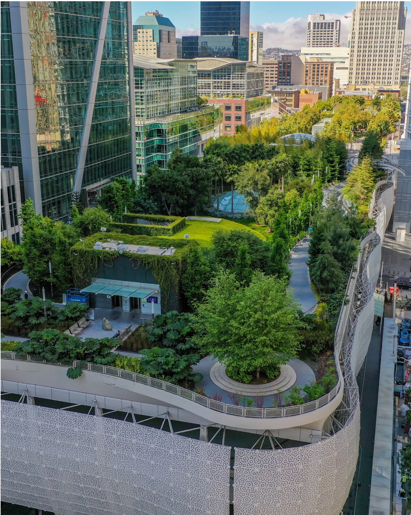
PHOTO: The rooftop green space of the Salesforce Transit Center offers an urban hideaway.
