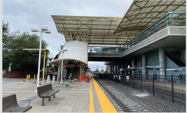
Southbound Caltrain platform at Millbrae Station
