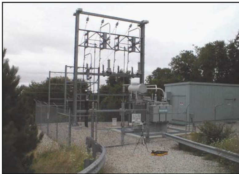
Figure 2-27 Paralleling Station
