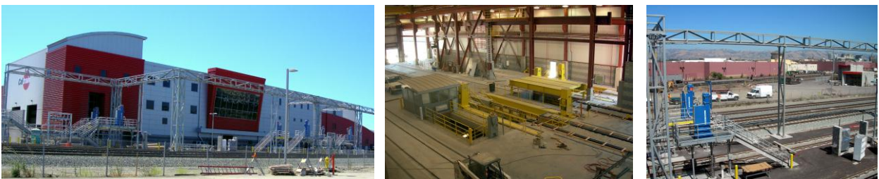
Caltrain SJ Maintenance Facility –Caltrain Graphics – Interior Repair & Exterior Fueling/Washing Area
