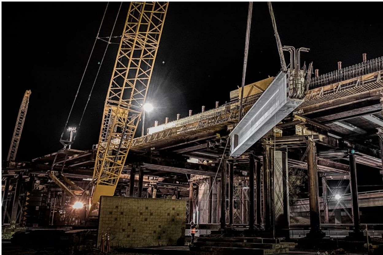
Photo: Nighttime girder at the Cedar Viaduct
