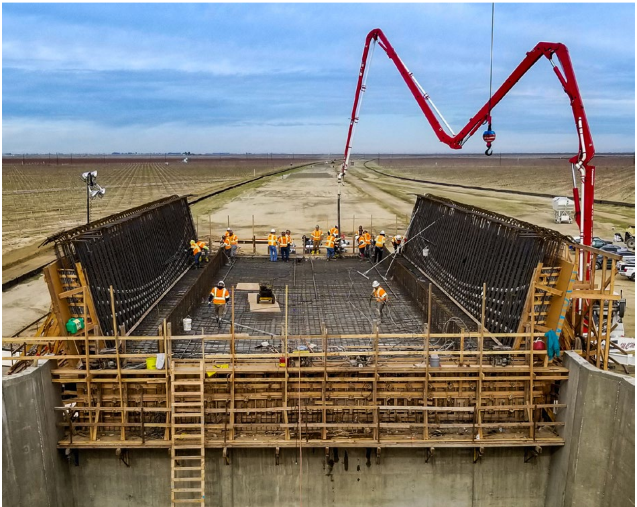
Photo: Construction at Garces Highway Viaduct
