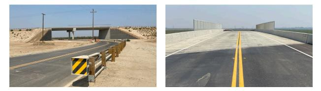
Work at the Avenue 7 overpass included straightening out a bend in the road and realigning Road 33, which travels underneath the structure. The overpass will allow traffic to travel over the future high-speed rail line. The structure spans more than 196 feet long, 43 feet wide and reaches 44 feet at its highest point.
