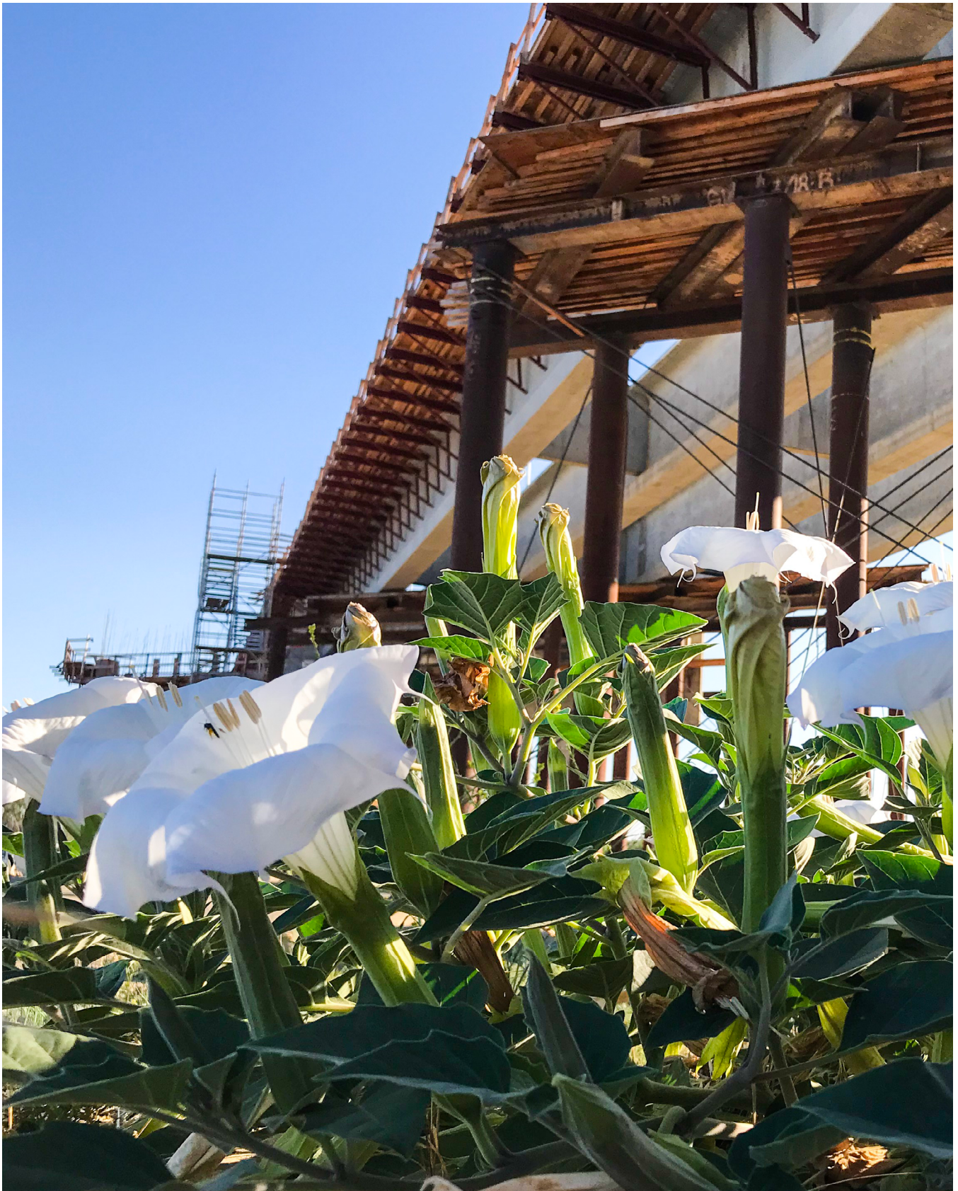
PHOTO: Flowering Datura under the viaduct construction at Road 27 in Madera County on the high-speed rail alignment.
